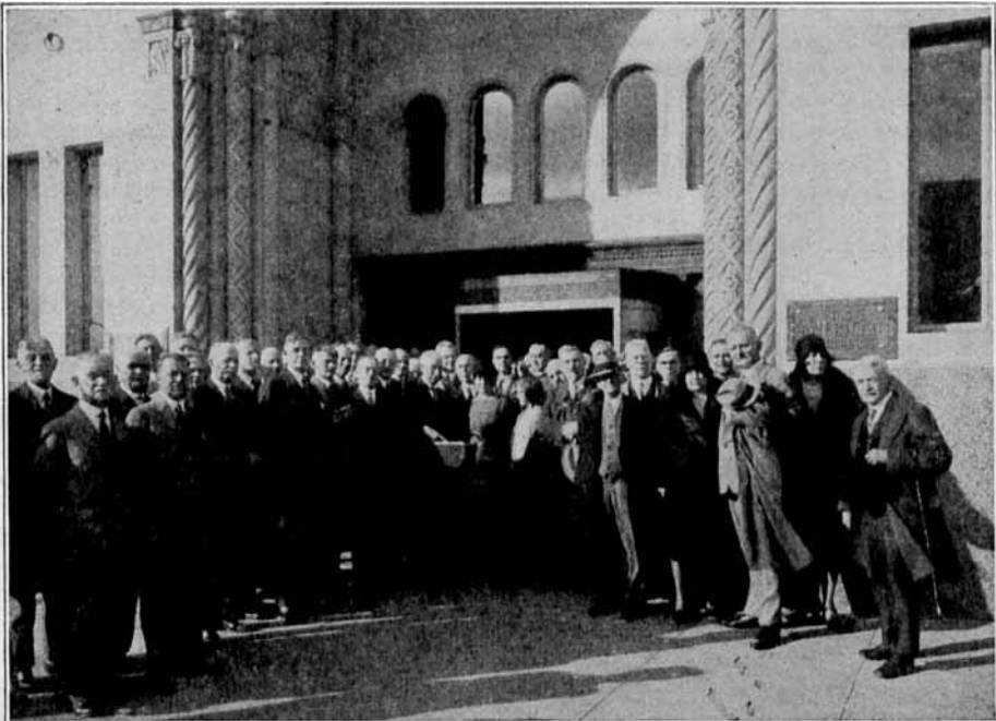
Filling the Century Box of the American Building.
